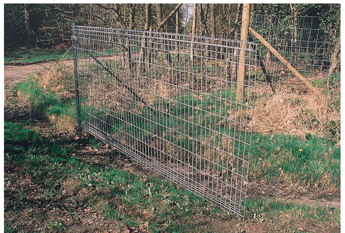
Figure 8 Rolled-top gate hung on T-bars
